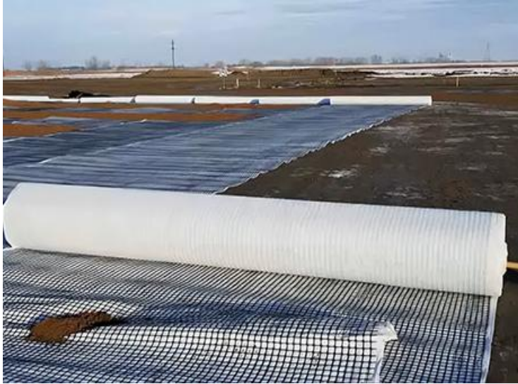
[Airport subgrade reinforcement in Sudan]
